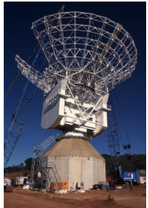
The framework of the new ESA 35m antenna being built at New Norcia (Australia)
